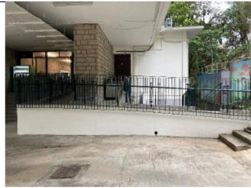
The ramp in the main entrance of canteen
