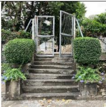
Steps from the drive to basketball courts
