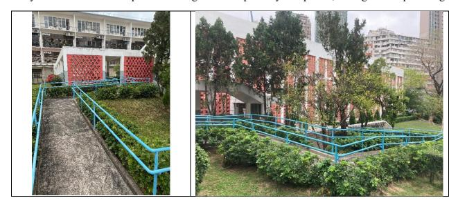
First, the ramp besides St. Ignatius Chapel has a gradient less than 1:12 and width of at least 1.05 m. Also, the ramp has provided with horizontal platform for every 10 m of inclined roads, which fulfils the safety regulation in Hong Kong.
